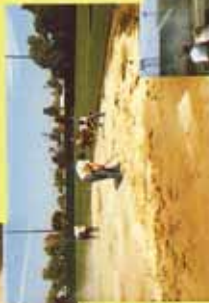
Spread with back of rake — 1/8"-1/4" thick. Allow to stand several minutes.
