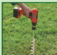
3. Mark and drill holes for poles with optional 18" auger.
