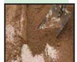
Step 3: For best results, make sure that the trench has at least a 1% slop from beginning to end. A 25 foot long trench would have a pitch of at least 3 inches (25 feet x .01 = .25 or 3 inches).
