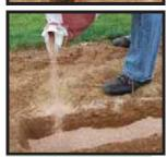
Step 1: Determine the number of trenches you will need for your area and mark out placement. Every inch of depth in your trench, water will be pulled from 1 foot on either side of the trench. A 6 inch deep trench would require a trench every 12 feet. However, a trench a few inches in from the grass edge of a skinned infield will provide excellent drainage.
