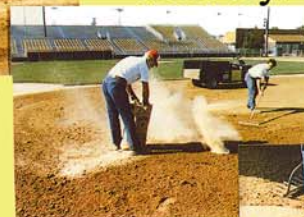
Top dusting the remaining damp spots.
