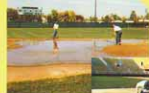
Remove excess water.
