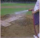
STEP 4: Once the BRICKS have been placed, water the cut area. Tamp the BRICKS into place.
