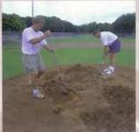
STEP 2: Cut out and remove all loose dirt from the high stress area surrounding the pitcher's mound to a depth of 3".
